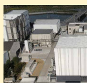
Overall view of the plant and office building completed in FY2022
